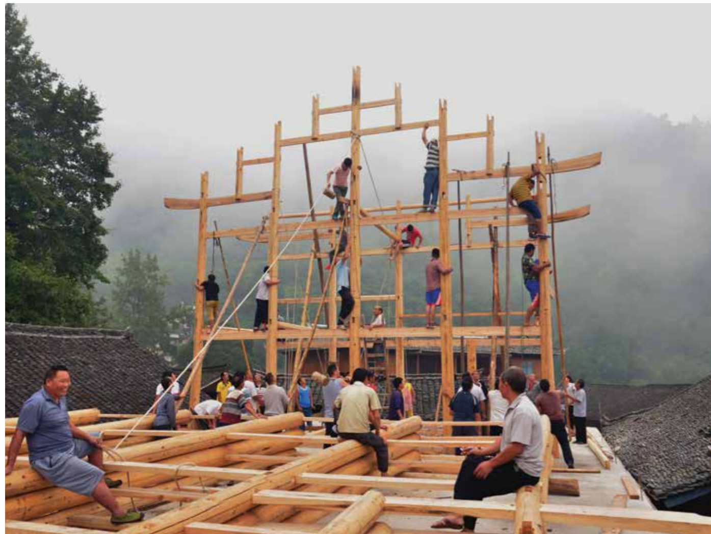
Building house 起房子
