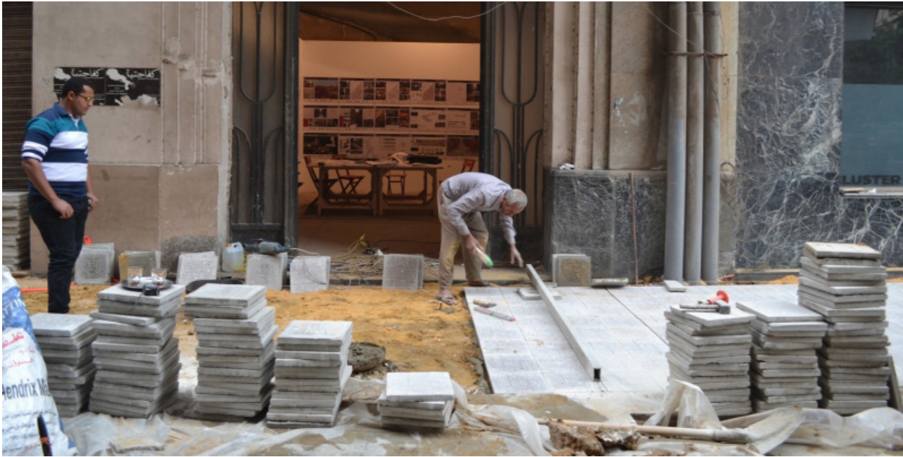
Fig. 22 The Kodak Passageway under renovation 8
