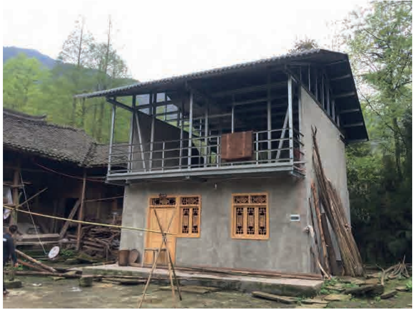
Steel, recycled stones and wood are integrated. 钢构与回收石材、木料结合使用。
